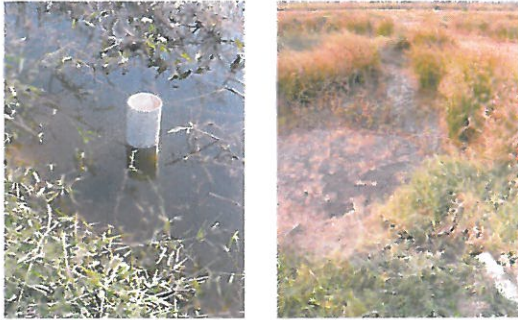
Dry season water management – uPVC pipes to control levels
